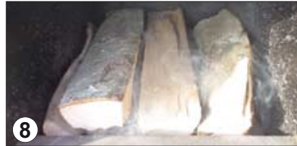
8 Completely close the bottom door and fill upper fuel chamber with logs.
