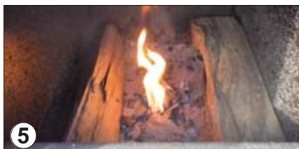
Position 2 wood logs on each side of the boiler wall
